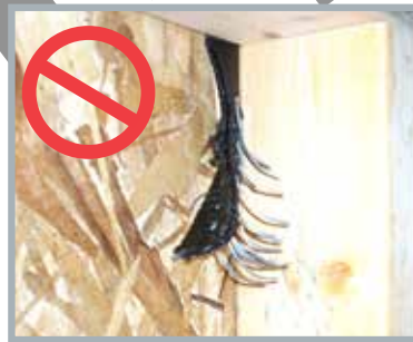
Figure 1: Unacceptable strap and attachment damage
